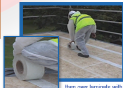
...then over laminate with glass fibre bandage tape.
