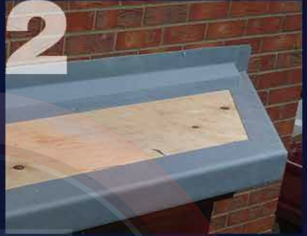
Stage Two Edge Trims Fitted
