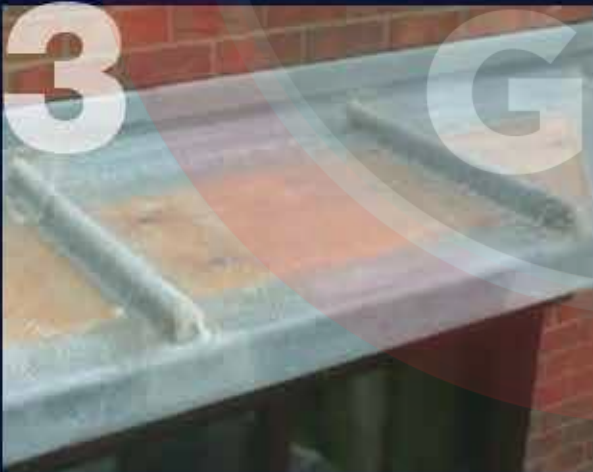
Stage Three Lamination and Cure
