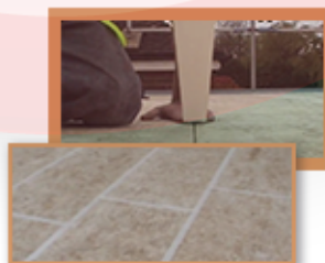
Cover joints with 25mm masking tape...
